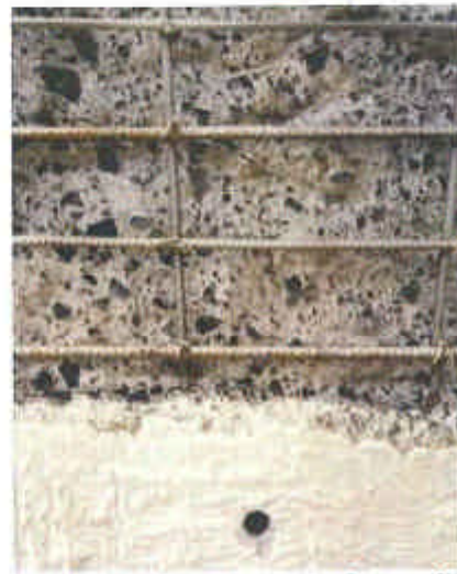
Figure 5 – Concrete surface after preparation, ready for concrete spraying.
