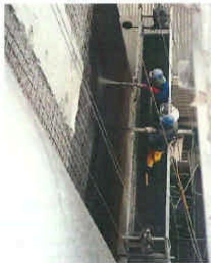
Figure 6 – Concrete spraying.
