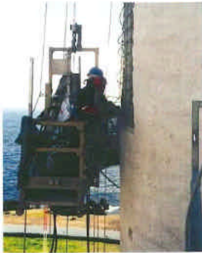
Figure 4 – Removal of deteriorated concrete.
