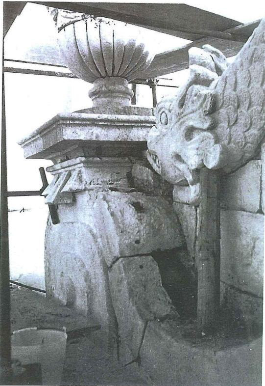
**Before Restoration :** "black crusts" formation consequent to the sulphatation phenomena with englobation of atmospheric polluting microparticles.
