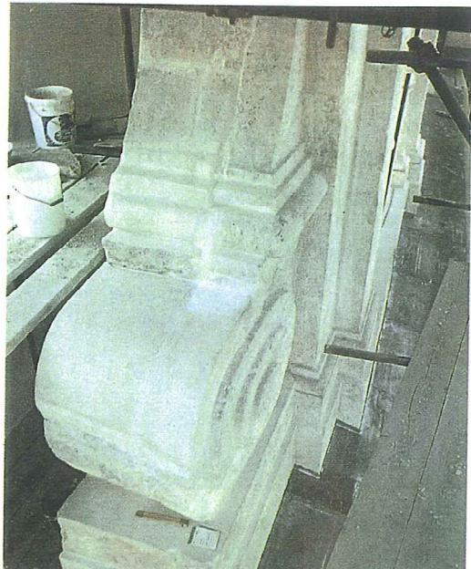
**In course of Restoration : microcracks and cracks sealing and partial reconstruction of missing parts have been executed using Spartyte® MAR GRIP ZB, different versions according to chromatic tonalities needed.**
